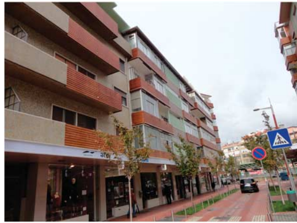
Figure 11: Av. Santos Mattos. Detail of the new street pavement and commercial gallery.
