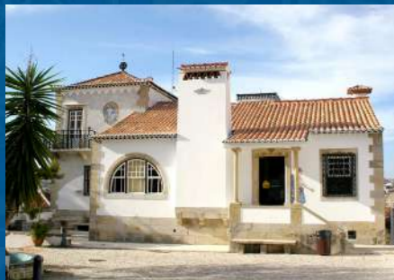
Southern facade of Casa Roque Gameiro, 2016. © Luísa Baeta
